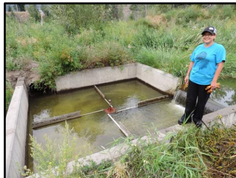
4. The Finnegan Screen: current enters in the lower right corner; the bypass taking smolts back to the creek is in the upper left corner.
